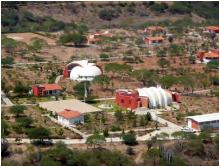
University of La Cañada. Partial view from the air.
